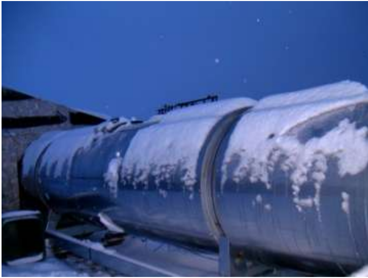
Photo 4, December 16, 2005: Exterior installation.
